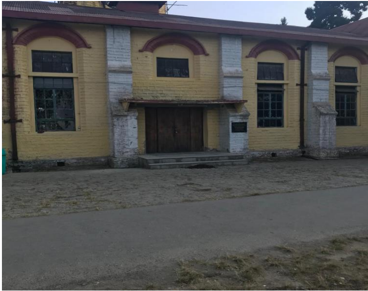
Roof Repair and Painting in progress – Apr 2024
