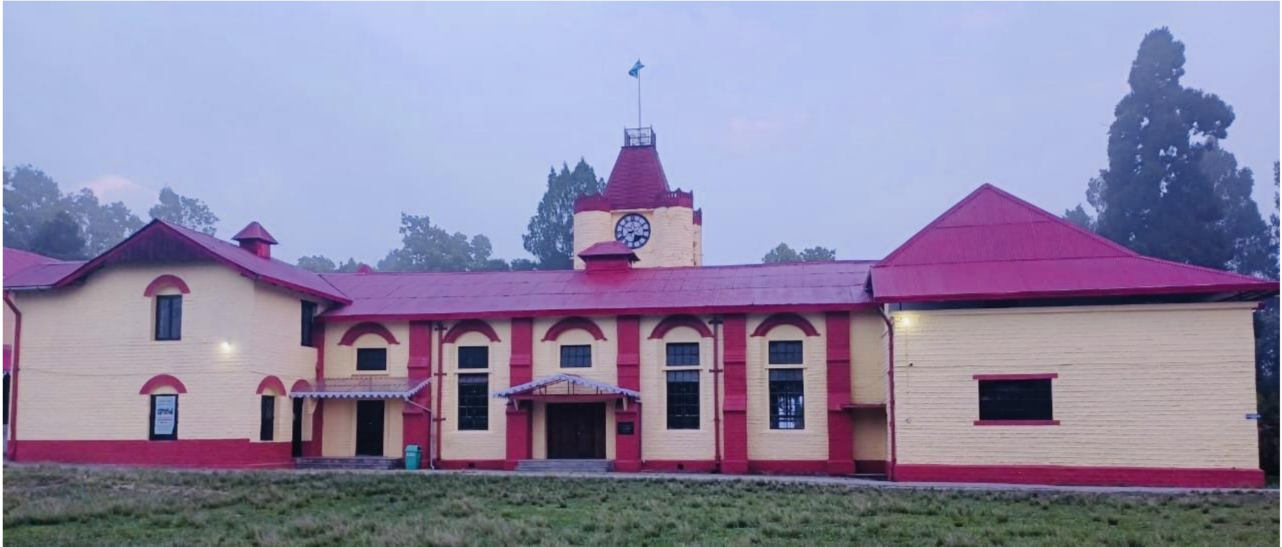
New awnings installed above the 2 doors entering the Hall – May 2024
